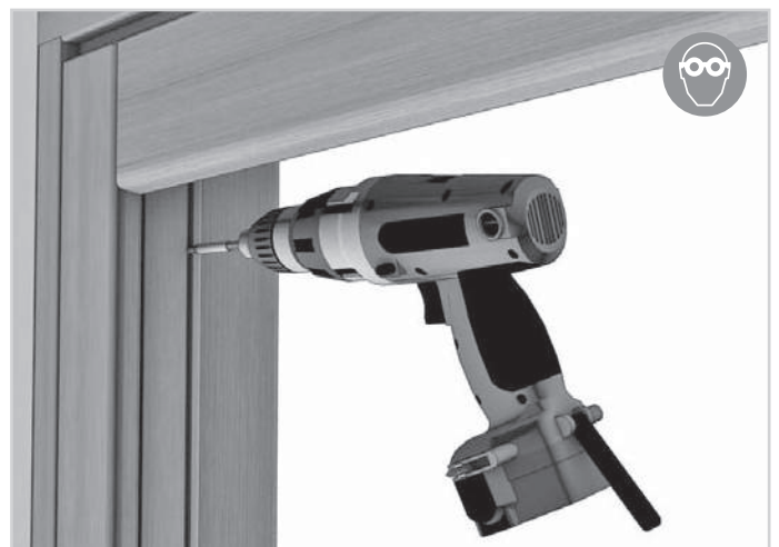
66. Pre-drill holes diagonally under the glazing bead.
