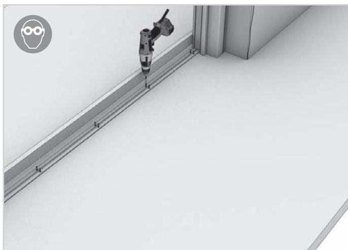
27. Secure with 3,5x40 mm screws.
