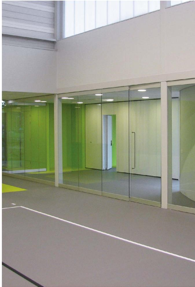
Our Flexirol Multidirectional Glass is a bespoke system for glass panels weighing up to 500kg and requiring 90 degree or 135 degree movement. When open, panels stack neatly to one or both sides of the opening, leaving the walkway clear of obstruction.
